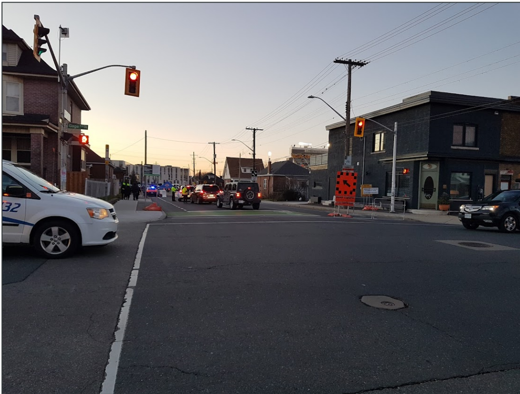
Figure 6 – Example of a Soft Closure
