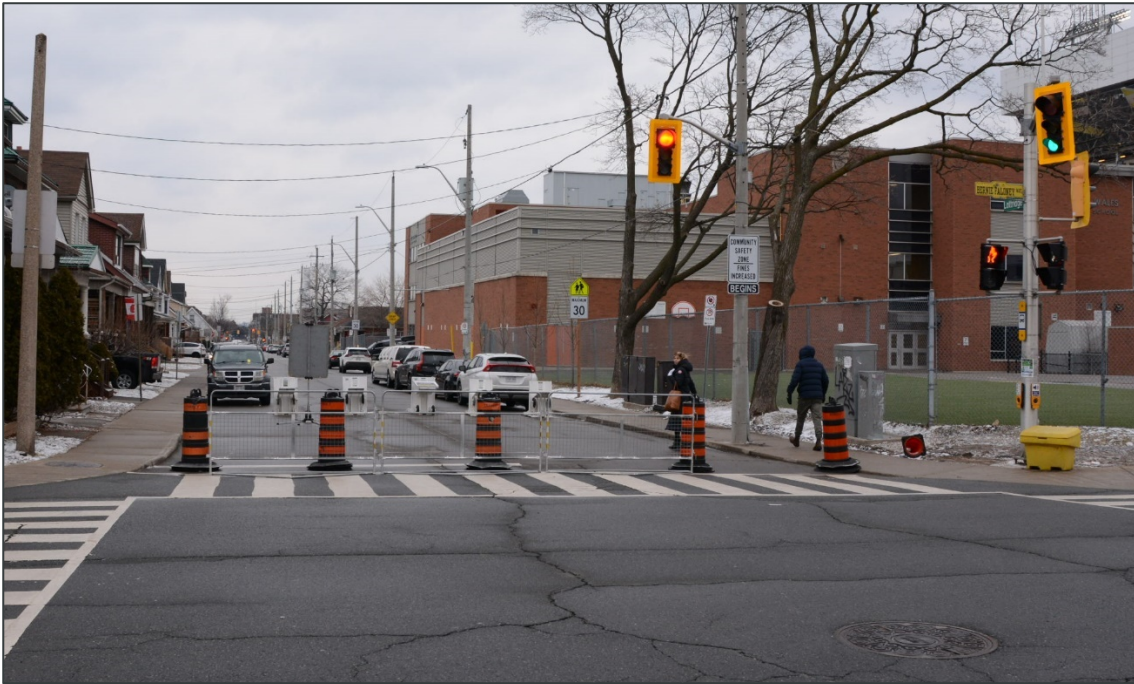
Figure 7 – Example of a Hard Closure
