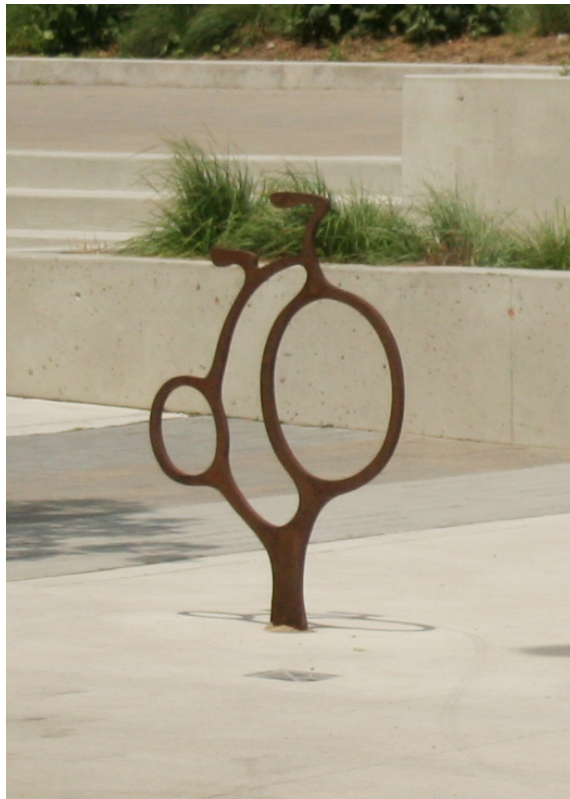
Penny-farthing bike rack constructed out of weathering steel (designed/manufactured by Artist Scott Eunson)
